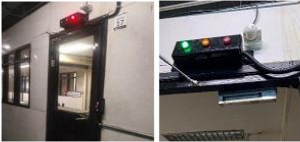
Figure 5. Installation of Warning Indicator Lights.
