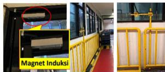
Figure 4. Installation of Mechanical Sensor and Magnet.
