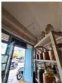
Business Area Store room located at the front of the building
