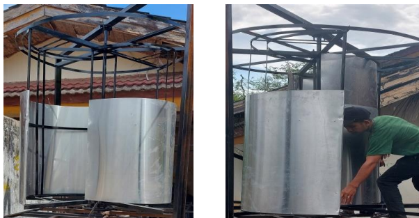
Figure 2. Assembled the turbine rotor blades
