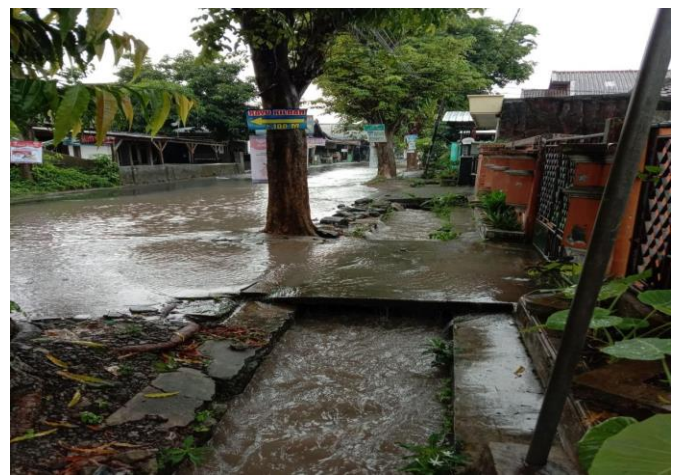
Fig. 2. Flood in local residential area due to improper drainage system
