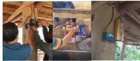
Fig. 6. Installation of SCC Control, Inverter, and Battery
