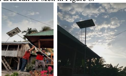
Fig. 5. Installation of solar cell panels
