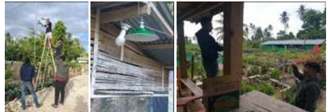
Fig. 7. Installation of cables and lights in the fish pond area
