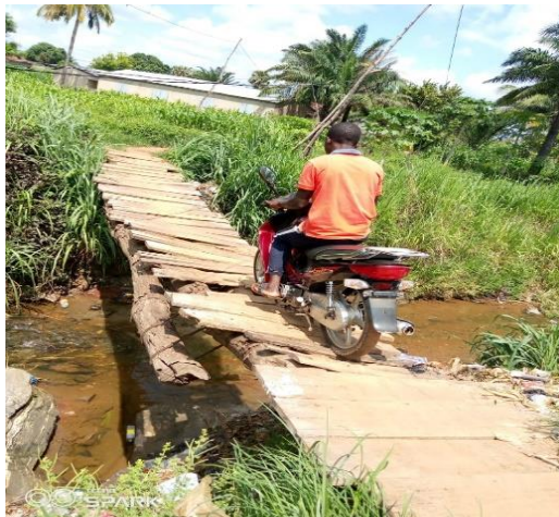
Source: Photo AGBAMARO, October 2021 Photo 2: A wooden culvert over an alley in Eyéouda
