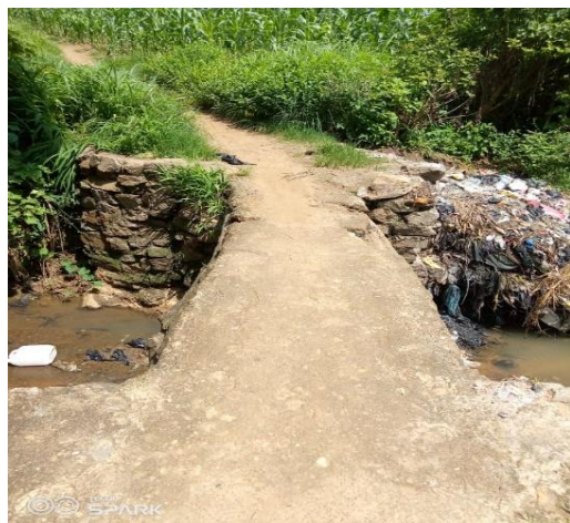
Source: Photo AGBAMARO, October 2021 Photo 3: Crossing scupper at Tchintchinda
