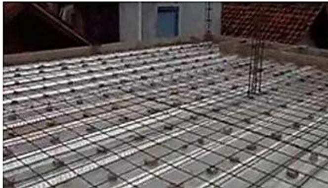
Fig. 3. Steel deck Floor Plate and wiremesh installation
