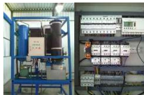
Figure 5. Modification of ice machine and smart relay control panel results
