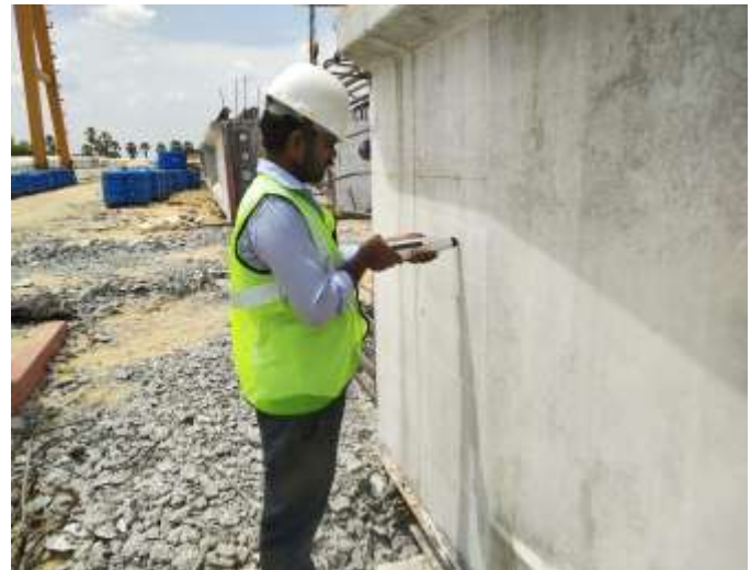
Fig. 2. Photo 2 shows a view of the Rebound hammer test in progress in a PSC Girder.
