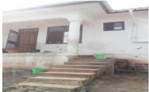
Fig. 4. Steep steps on the entry way inhibiting free passage at house level.
