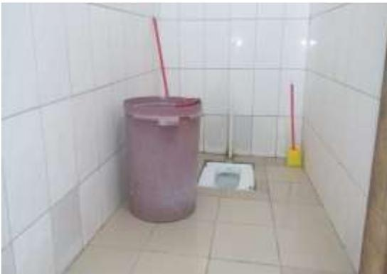
Fig. 9. Combined bathroom and toilet without hand support fittings.
