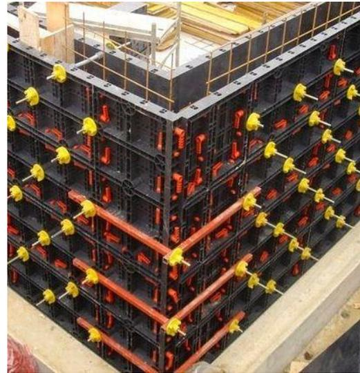
Plastic formwork concrete wall
