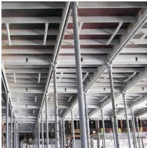
Aluminum shuttering in roof slab casting
