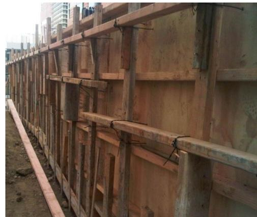
Plywood forms in combination with timber
