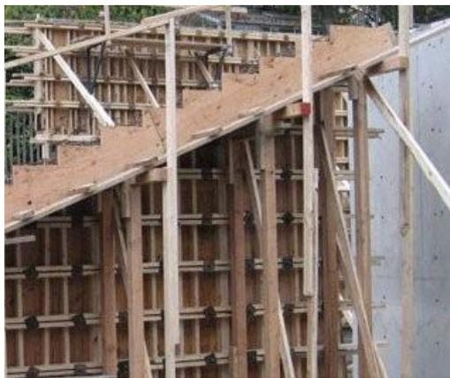
Timber formwork in staircase construction
